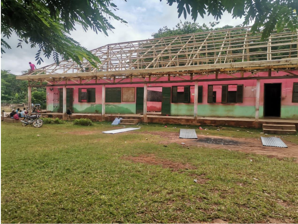
RENOVATION OF NKRANKWANTA D/A JHS
